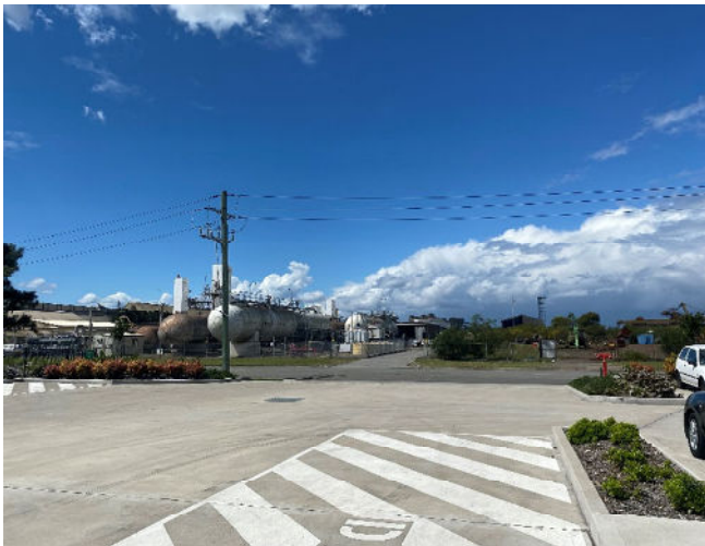
Photo 7: Photo of the entrance into site.
