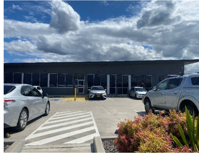
Photo 2: Looking towards the entrance of the facility, featuring the car park.
