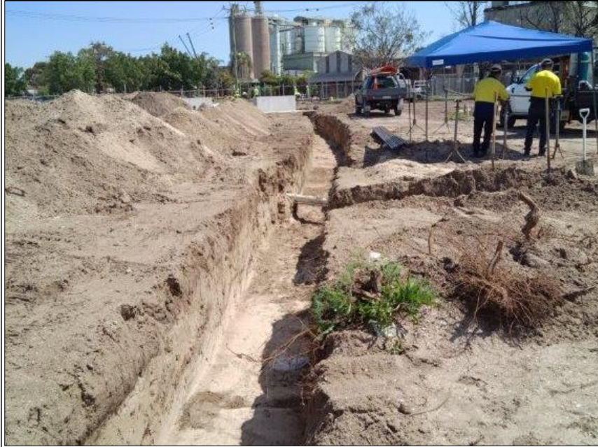
PHOTO 2 – TRENCHING FOR INSTALLATION OF ELECTRICAL SERVICES
