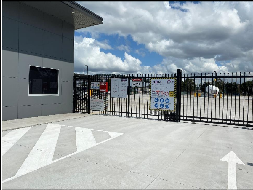
PHOTO 4 – VIEW OF STORAGE AREA AT COMPLETION OF CONSTRUCTION
