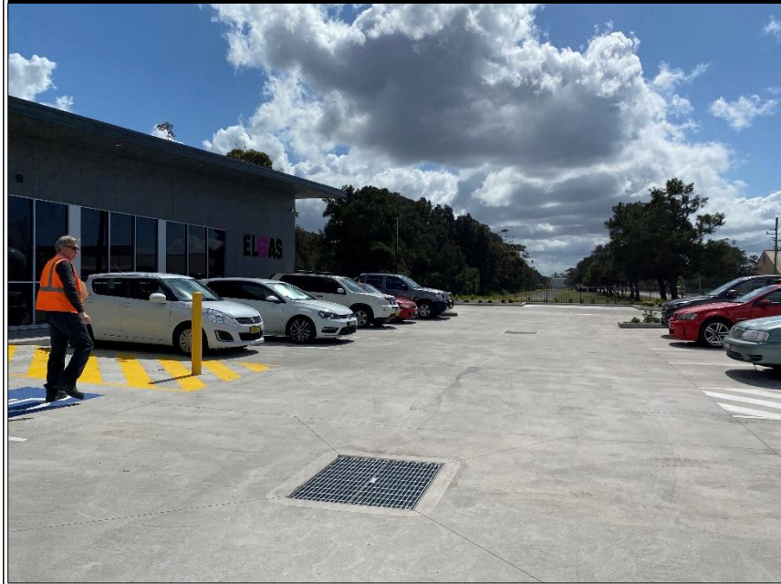
PHOTO 6 – COMPLETED CARPARK AND STORMWATER DRAINAGE PIT
